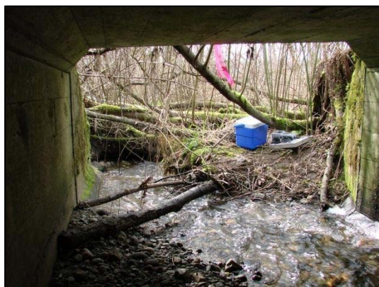
Figure 20a. Drainage channel upstream site at SR203 crossing. SCD photo March 2007.
