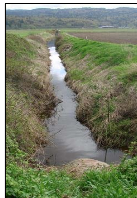
Figure 20b. Drainage ditch downstream site. SCD photo April, 2007
