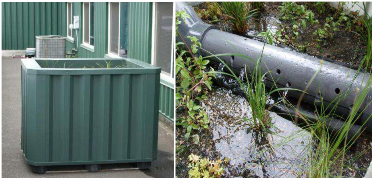
Figure 3. Roof drain using biochar for filtering zinc from roof runoff. (Miles 2010, http://www.futureenergyconference.com/2010/FECWA-Presentations/4D_Miles.pdf ).
