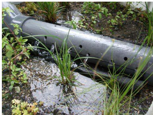
Figures 3 and 4. Roof drain using Biochar for filtering zinc from roof runoff (From Tom Miles, Washington Future Energy Conference 2010.)
