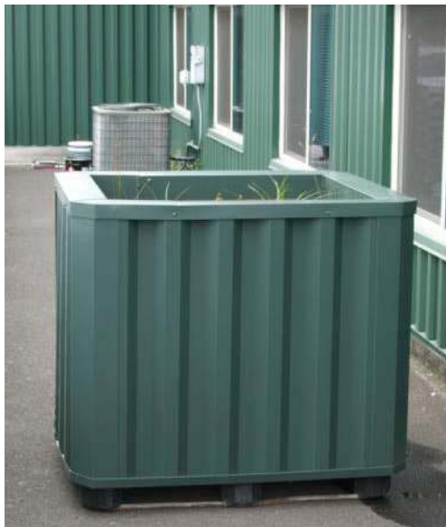
Figures 3 and 4. Roof drain using Biochar for filtering zinc from roof runoff (From Tom Miles, Washington Future Energy Conference 2010.)
